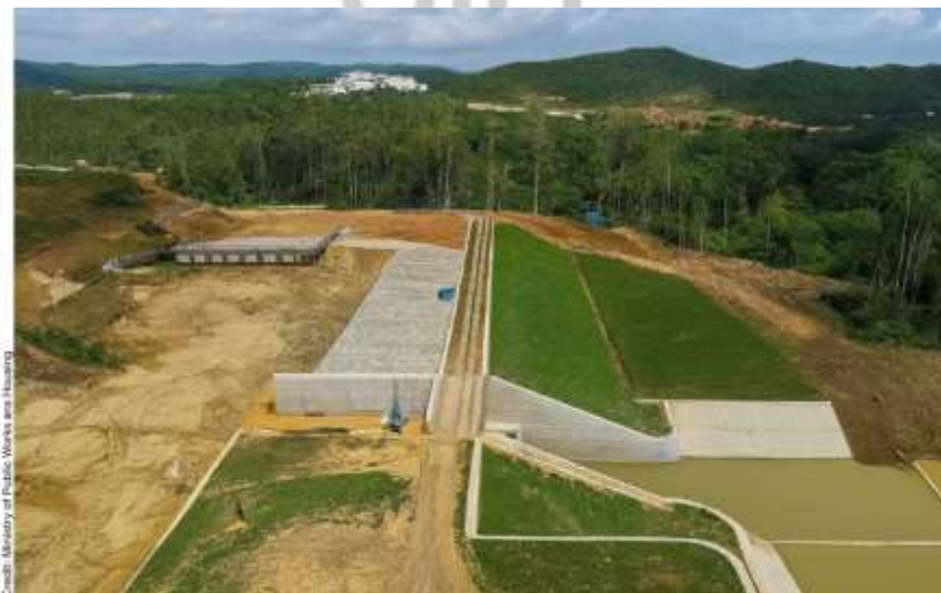
Gambar 1. 2 Pamaluan River Flood Control Project comprises river normalization, embankment construction, and drainage rehabilitation.
