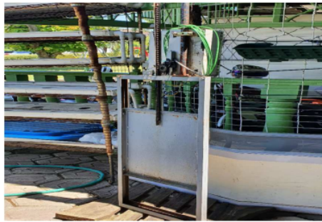
Fig. 10. Implementation of watergate system.
